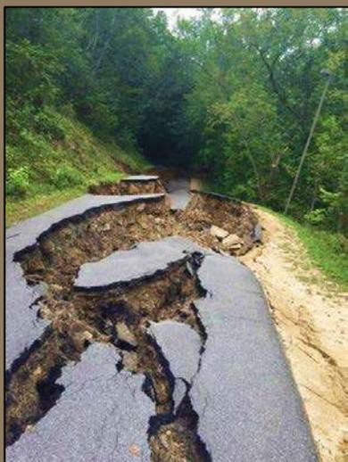
August flood waters did a lot of damage. The Dug Road portion of Trout Run Trail suffered a major landslide and is closed indefinitely.
